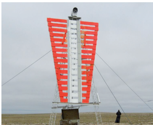
Leading (Rear Range) Light - Photo Courtesy of the Canadian Coast Guard
