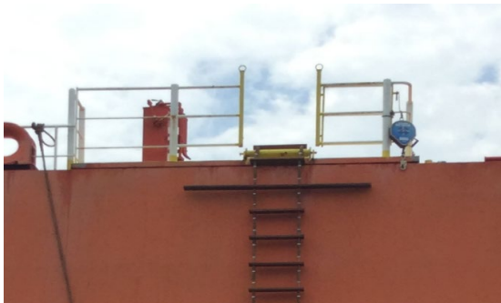
Figure 2: Gap in handholds appear to accommodate spreader.
